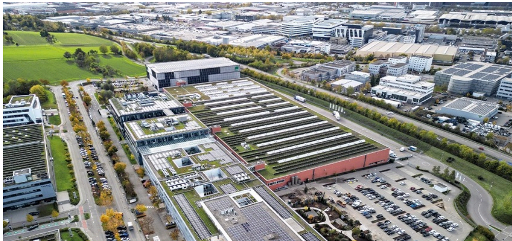
The Bechtle Group headquarters in Neckarsulm scores highly as a sustainable location: over 7,000 solar modules on all available roof surfaces, 261 geothermal probes underneath the office and warehouse buildings, building technology with natural coolants or 7,500 square metres of green space. Copyright: Leo Dörfele
